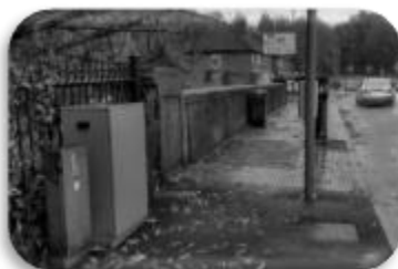
Path width reduced by bollards and posts
