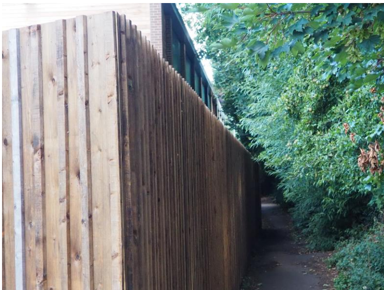
Dark & uneven surface. Deterring users.
